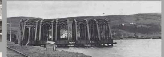
New train bridge spans assembled in 1915.
