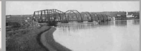
The original train bridge that was built in 1890.
